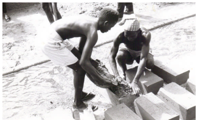
Making concrete blocks for the walls
