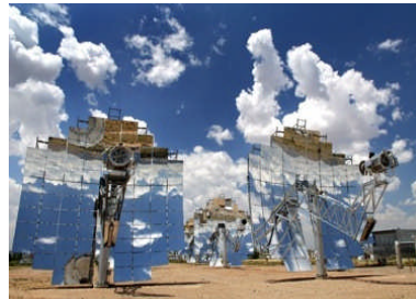
Dish System uses a large sun-tracking mirror with a Stirling engine generator at its focal point to convert heat energy into electricity.
