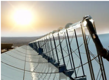
Trough Systems use parabolic trough shaped mirrors, each one of which focuses light on to a tube containing oil or similar fluid that takes the heat to where it can be used to raise steam and generate electricity.
