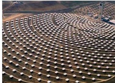
Power Towers use a large field of sun-tracking mirrors to concentrate sunlight on to a central receiver on the top of a low tower to raise steam and generate electricity.
