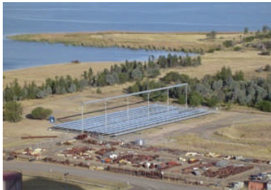
Fresnel Mirror Systems are similar to trough systems but use long flat mirrors at different angles to concentrate sunlight on to a tube containing heat-collecting fluid.
