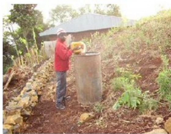
Water for construction poured into tank
