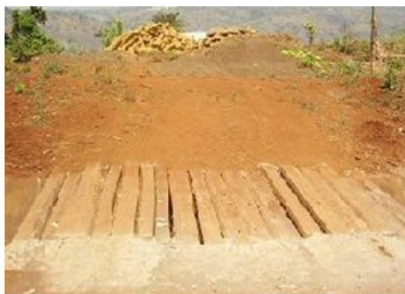
Planks laid across highway ditch
